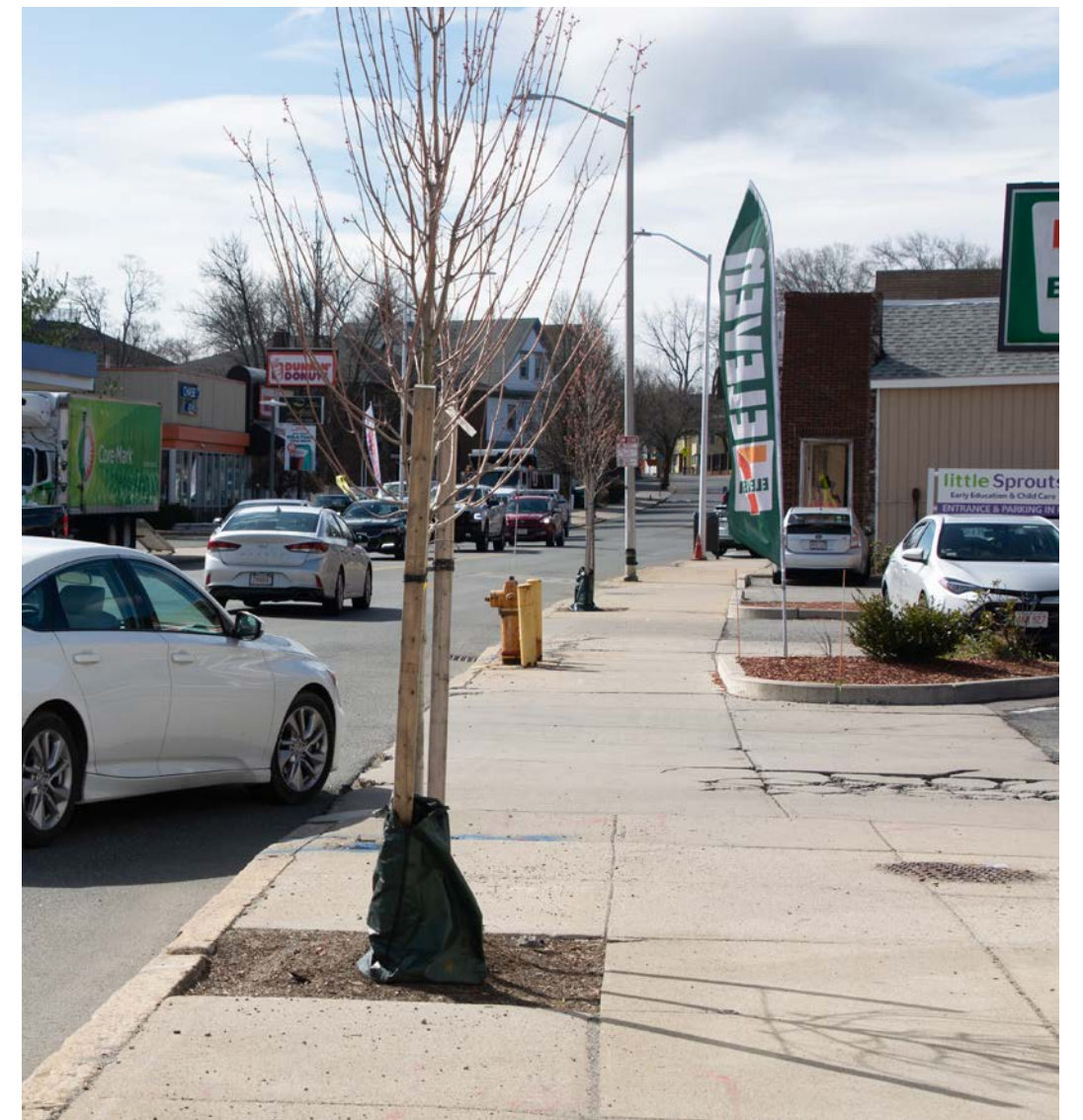
Figure 4 SeeClickFix tracks resident requests to understand patterns of deferred maintenance needs.
