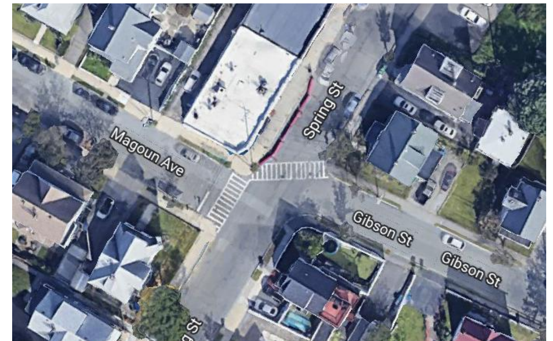
Figure 4. The corner of Spring Street and Magoun Avenue
