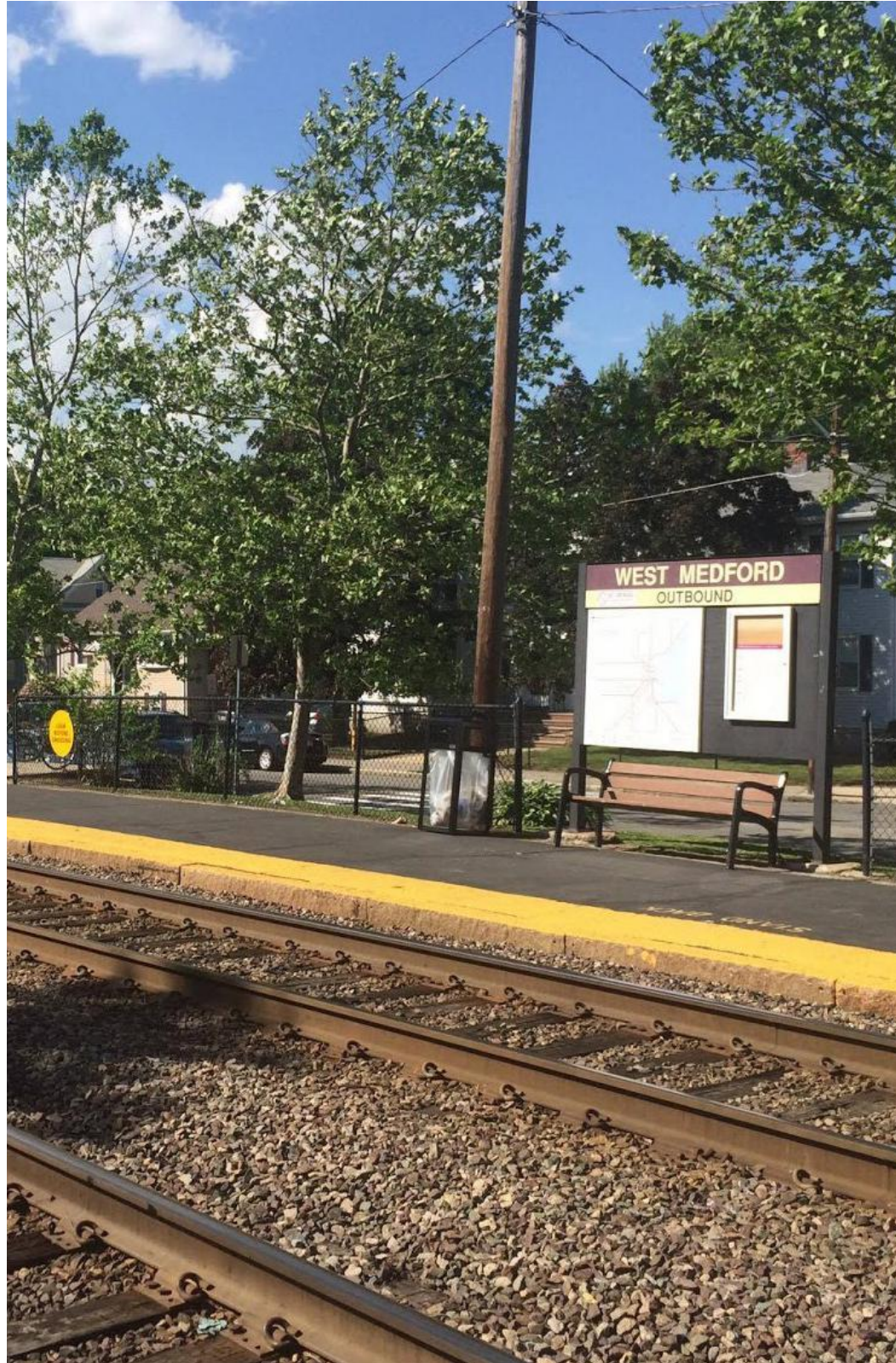
Figure 14. The West Medford station is currently in need of universal accessibility updates for persons with physical, hearing, and visual impairments.
