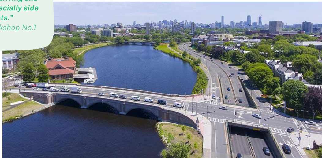
Figure 5. A city-wide infrastructure repair strategy prioritizes much-needed roadway investments in Medford.
