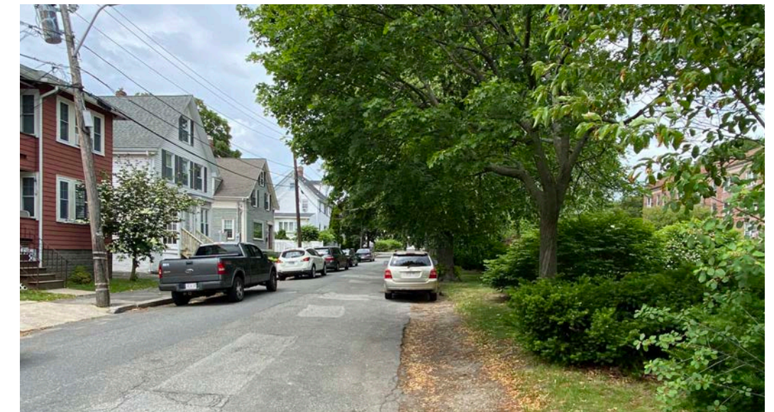
Figure 5. Street and sidewalk repair and maintenance are critical needs.
