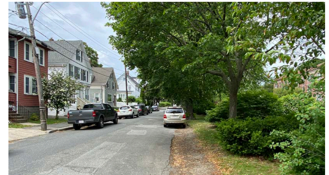
Figure 11. Street and sidewalk repair and maintenance are critical needs.
