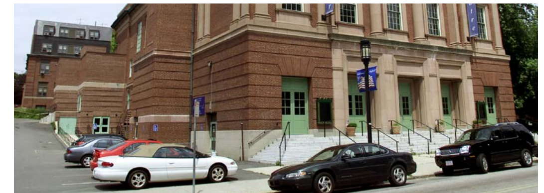
Figure 7. The need for clear parking strategies in Medford Square was a priority for community members during the third public workshop.
